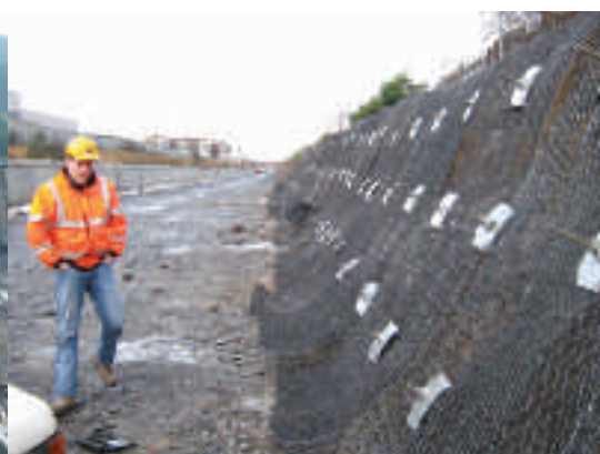
MacMat®R and Soil Nailing
