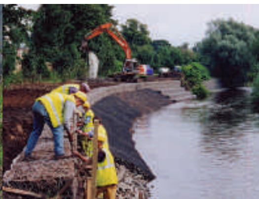
River Usk - under construction
