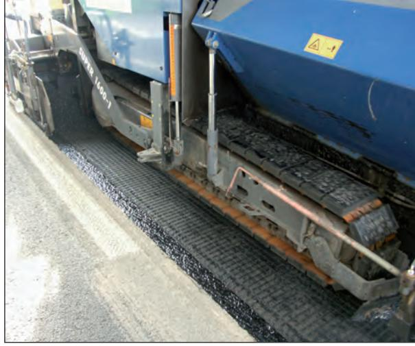
The reinforcement grid must be laid free of folds and waves. However, if a slight wave builds up in front of the paving machine, this will not detrimentally affect the performance of the reinforcement.
