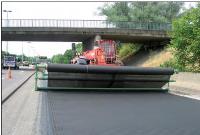
The unrolling can be undertaken with the help of a simple system, either manually, or mechanically when using wider, heavier rolls. The grid should be pulled equally on both sides of the roll, in order to prevent the development of folds and creases.
